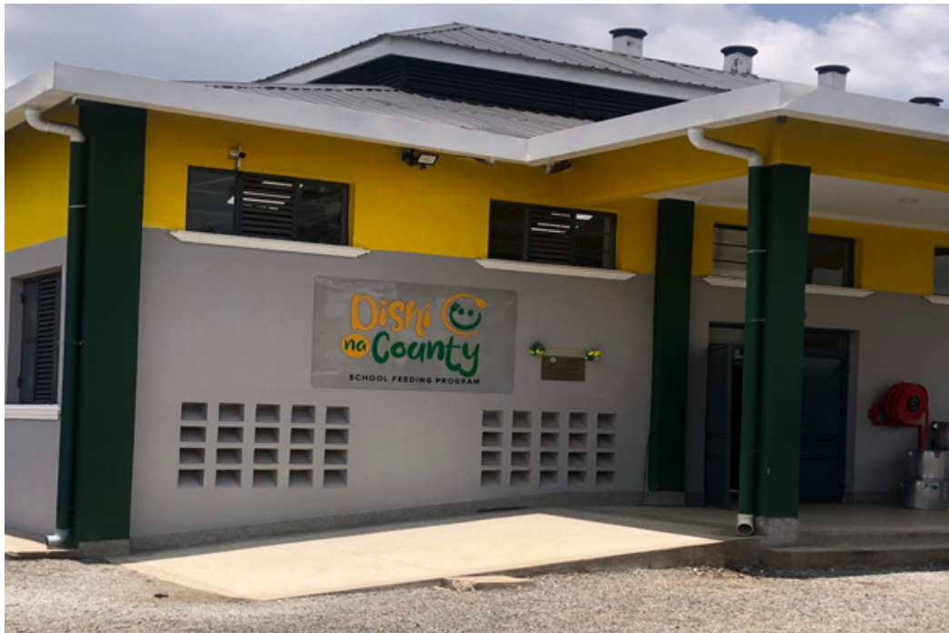
View of the recently launched Baba Dogo Kitchen, construction funded by the Nairobi County Government
